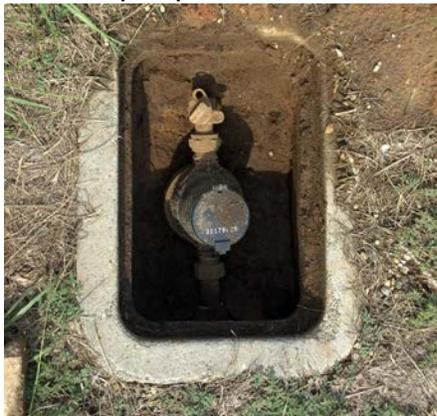
Step 4: On the face of the meter there is a large dial and a display of numbers. Read the number display from left to right (including any stationary or painted on numbers). This is your meter reading. The meter below reads 0000450 and your bill would show 000400 since we do not bill for the 10's or 1's.
